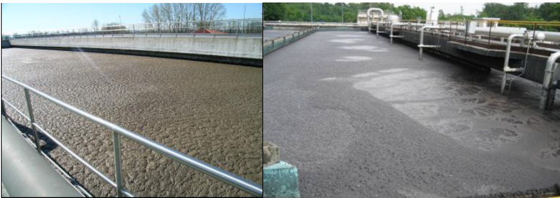
Figure 2: Foam on aeration tank in Lariana before (left) and during (right) ozonation [4]
